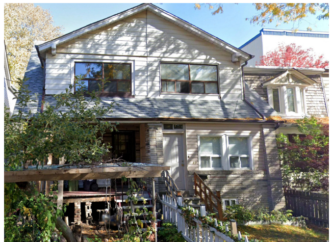
Photo 16: 9 and 11 Lewis Street Low-rise Residential Dwellings Along Lewis Street
