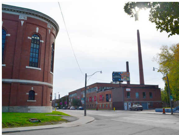
Figure 22: Carlaw Avenue looking south towards TOC site and corner of the Toronto Hydro Substation
