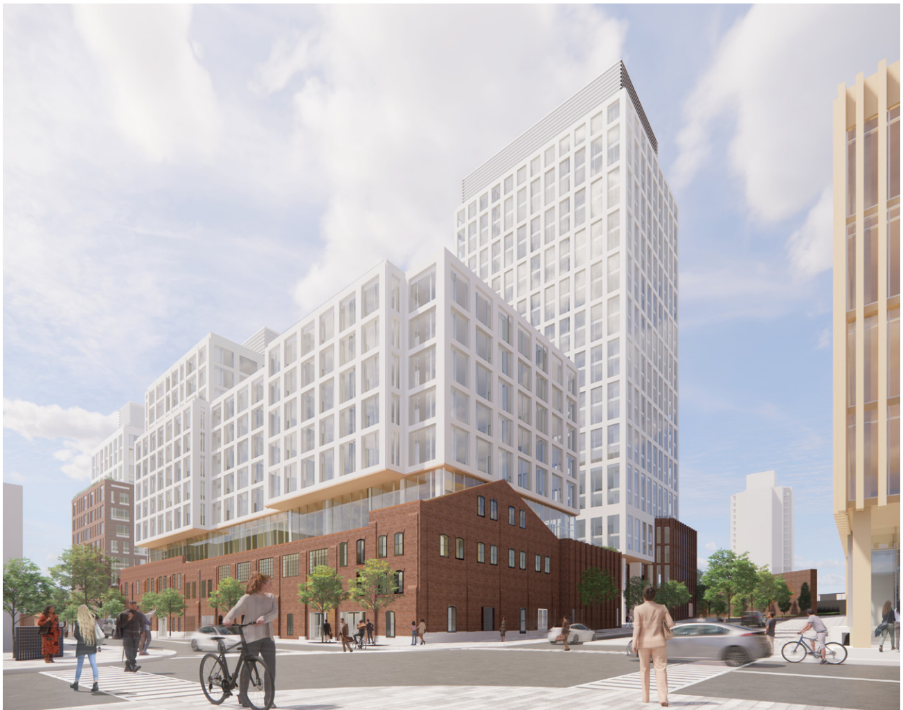
Figure 69: Artist's Rendering of the Gerrard Carlaw TOC from Carlaw Avenue & Badgerow Avenue intersection
