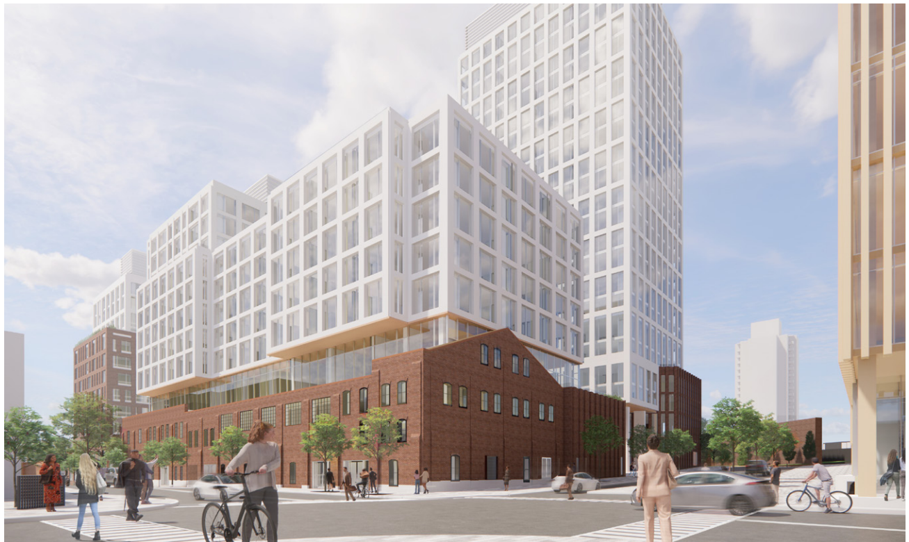
Figure 62: View of the TOC looking west along Carlaw Avenue
