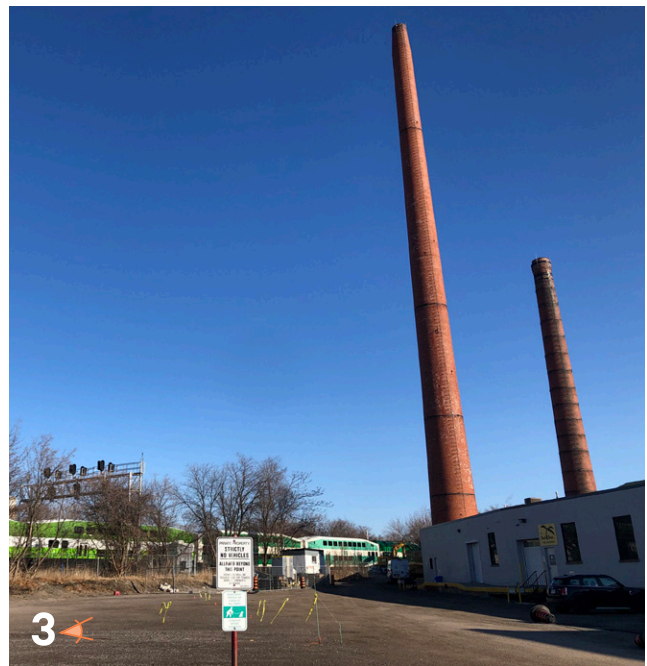
Figure 19: 388 Carlaw Avenue industrial chimneys located at the rear of the building
