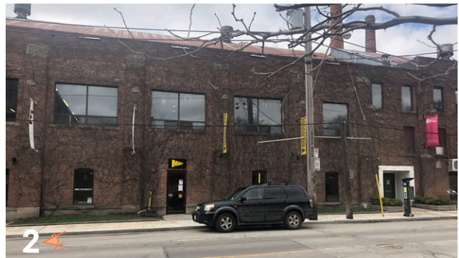
Figure 18: Portion of 388 Carlaw Avenue building façade
