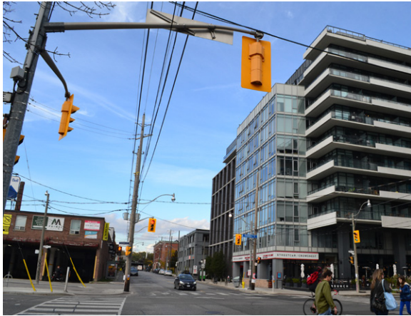
Figure 24: View north of Carlaw Avenue with mixed-use development at Dundas Street East (345 Carlaw Avenue)
