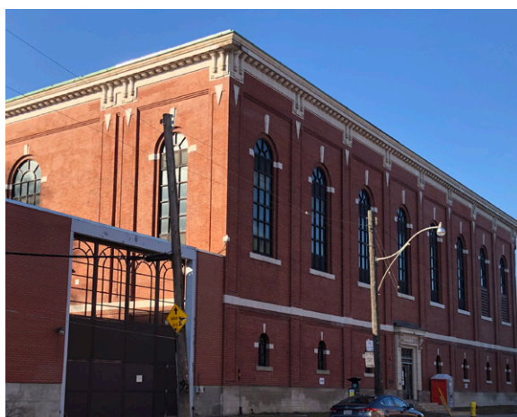
Figure 23: Toronto Hydro Substation frontage across from TOC site on Carlaw Avenue
