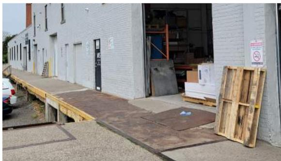
Figure 75. West elevation overhead door with corroded loading dock. Painted brick is deteriorated with extensive mortar loss on the upper portion of the wall (ERA, 2022).
