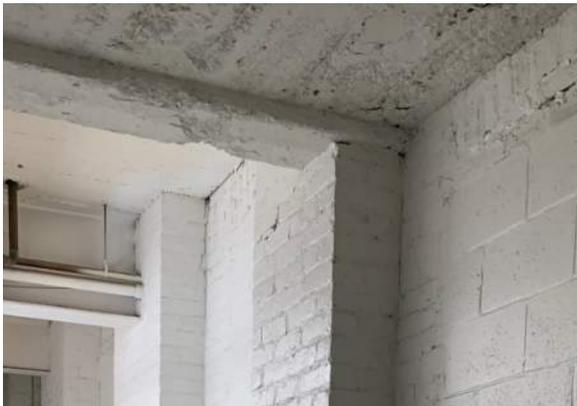
Figure 53. Concrete beam supports the concrete floor above in first floor hallway (ERA, 2022).
