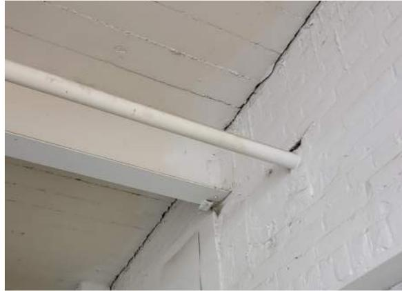
Figure 56. Separation of pier and slab from vertical wall at first floor along west side of 1912 portion of the building which may be due to structural movement (ERA, 2022).
