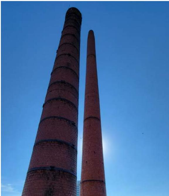
Figure 100. The shorter east chimney in the foreground with steel strapping, and taller west chimney beyond (ERA, 2022).
