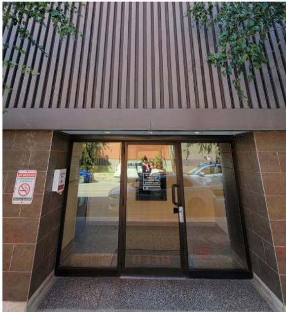
Figure 91. Main entrance with terrazzo floors and tile on exterior walls, and painted metal cladding above (ERA, 2022).
