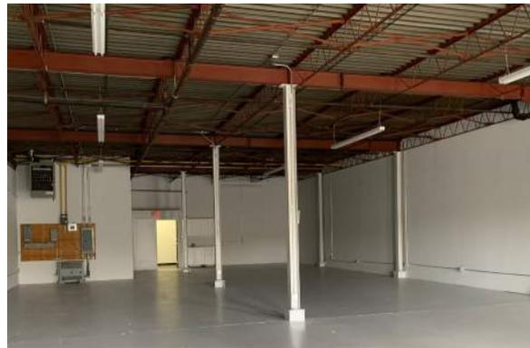
Figure 99. Steel columns connect to steel beams (ERA, 2022).
