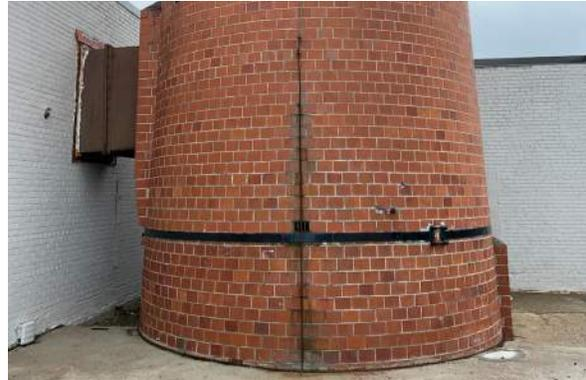
Figure 102. Taller west chimney exhibiting soiling, spalling and rusted steel tension bands (ERA, 2022).
