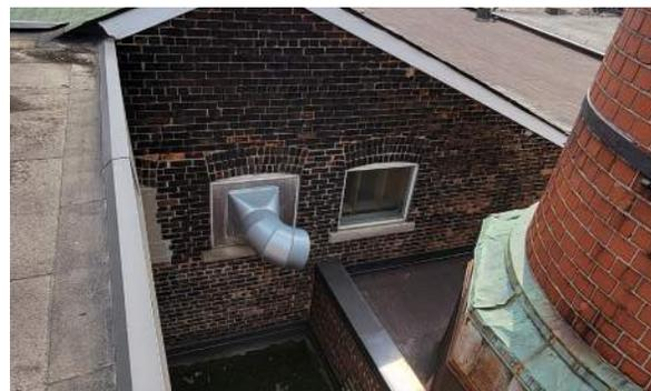
Figure 52. North gable brick wall with window infill and ductwork (ERA, 2022).
