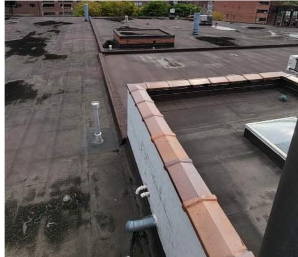
Figure 81. Flat roof sections with roofing membrane (ERA, 2022).
