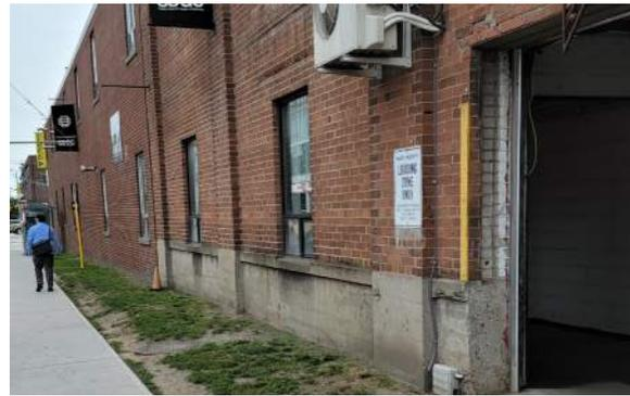
Figure 77. Brick piers separate each bay. Openings at grade have been modified for additional loading areas (ERA, 2022).
