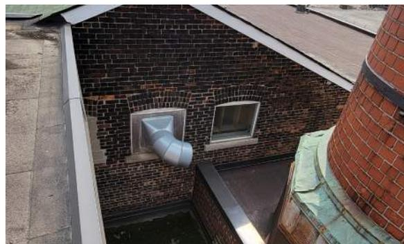
Figure 56. North gable brick wall with window infill and ductwork (ERA, 2022).
