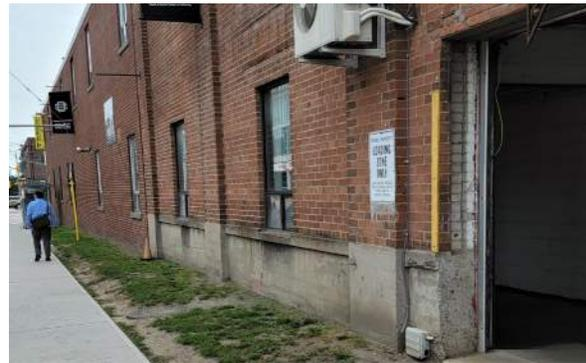
Figure 73. Brick piers separate each bay. Openings at grade have been modified for additional loading areas (ERA, 2022).
