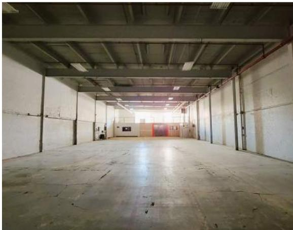
Figure 81. Looking west on second floor. This area has steel columns and painted brick (ERA, 2022).
