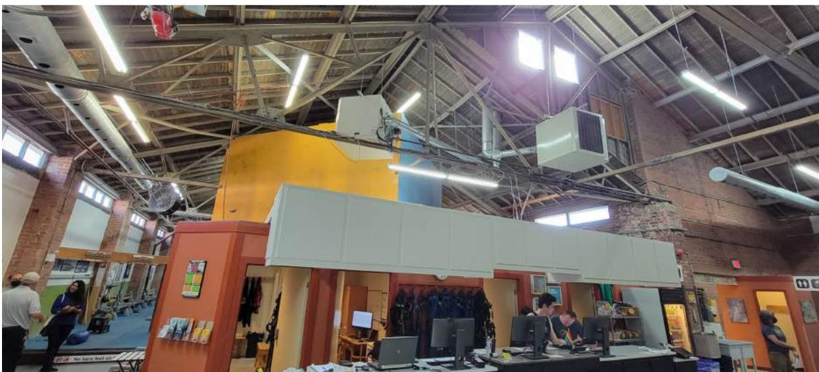
Figure 59. View of Unit 204 looking south, including steel trusses spanning east-west (ERA, 2022).
