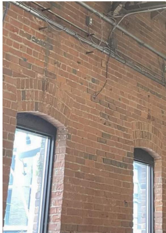
Figure 70. Window openings with segmental arch (ERA, 2022).
