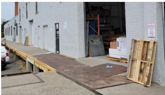
Figure 79. West elevation overhead door with corroded loading dock. Painted brick is deteriorated with extensive mortar loss on the upper portion of the wall (ERA, 2022).
