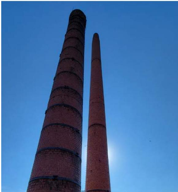
Figure 104. The shorter east chimney in the foreground with steel strapping, and taller west chimney beyond (ERA, 2022).
