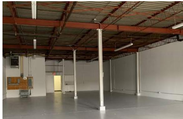
Figure 95. Steel columns connect to steel beams (ERA, 2022).
