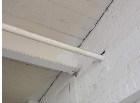
Figure 60. Separation of pier and slab from vertical wall at first floor along west side of 1912 portion of the building which may be due to structural movement (ERA, 2022).
