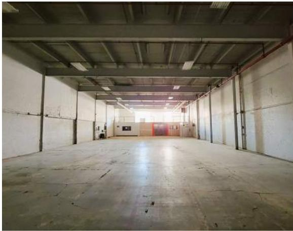
Figure 77. Looking west on second floor. This area has steel columns and painted brick (ERA, 2022).
