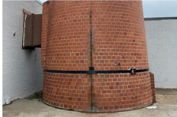
Figure 98. Taller west chimney exhibiting soiling, spalling and rusted steel tension bands (ERA, 2022).
