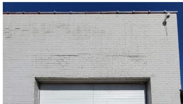
Figure 76. Brick spalling and mortar loss is evident under the painted surface (ERA, 2022).
