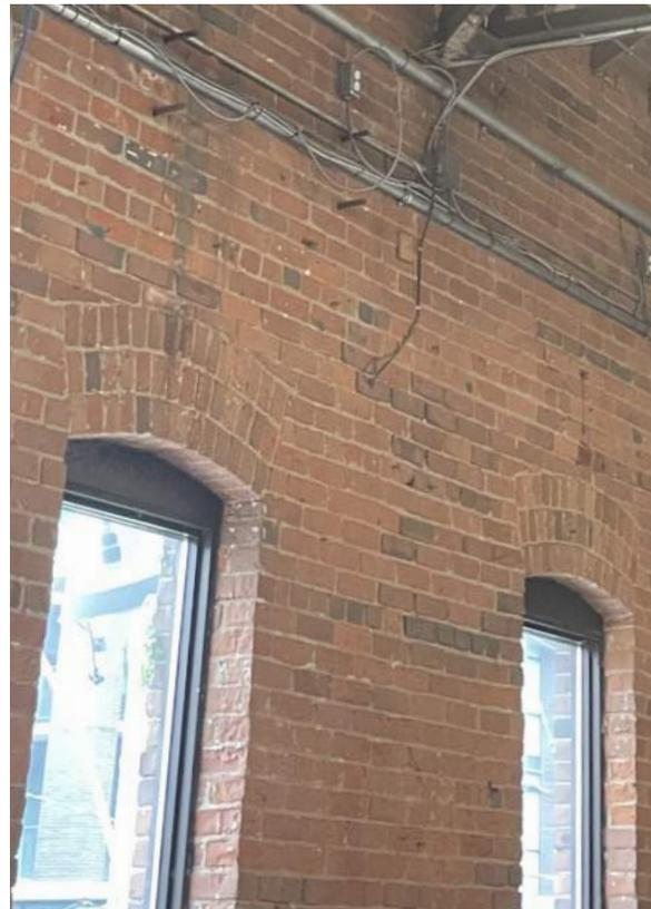
Figure 74. Window openings with segmental arch (ERA, 2022).
