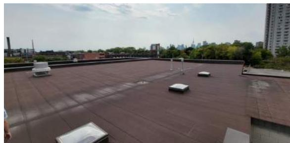
Figure 74. Roofing membrane with ponding and general deteriorated surface (ERA, 2022).
