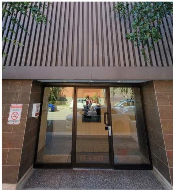
Figure 95. Main entrance with terrazzo floors and tile on exterior walls, and painted metal cladding above (ERA, 2022).
