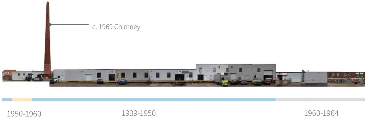
Figure 29. West elevation with approximate dates of construction (ERA, 2022).
