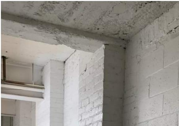
Figure 57. Concrete beam supports the concrete floor above in first floor hallway (ERA, 2022).
