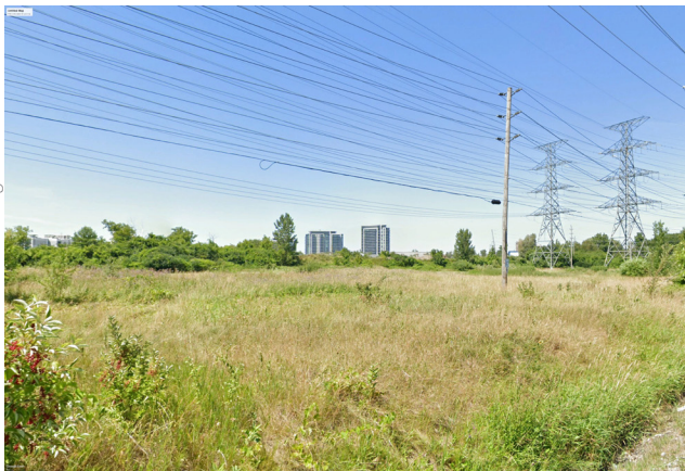
Figure 29: East York Hydro Corridor north of subject lands
