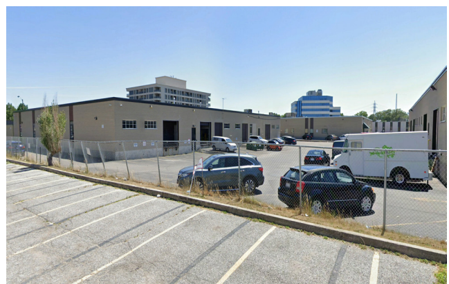
Figure 20: Rearview of 14-16 Overlea Boulevard, looking southwest
