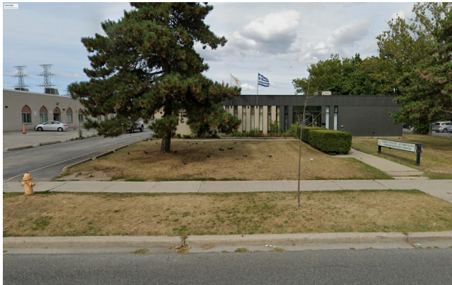
Figure 23: 6 Thorncliffe Park Drive looking east
