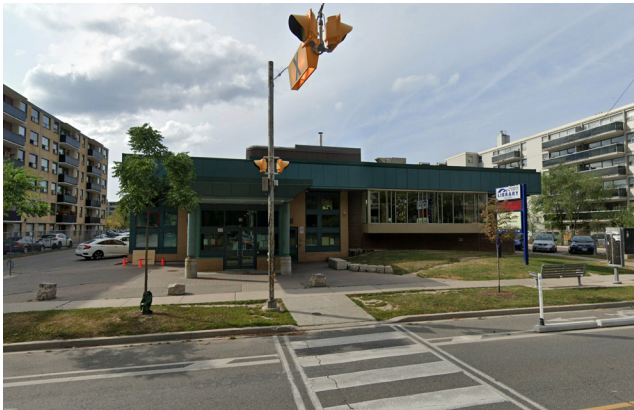
Figure 38: Thorncliffe Park Library at 48 Thorncliffe Park Drive
