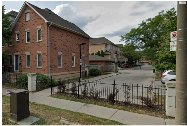
Figure 34: Townhouses to the southwest of subject lands
