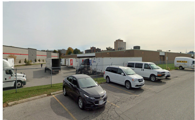
Figure 22: Rearview of 36 Overlea Boulevard
