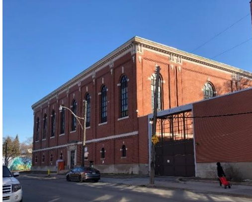
Toronto Hydro Substation frontage across from TOC site.
