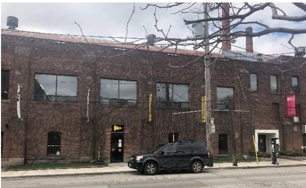
2. Portion of 388 Carlaw Avenue building façade
