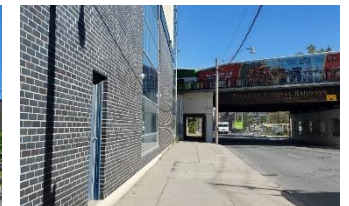
Eastern Avenue Underpass and Former Street Edge
