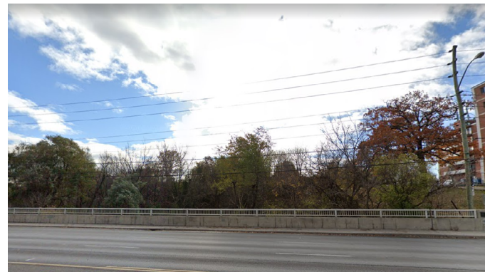
Lawrence Avenue Bridge over Highland Creek
