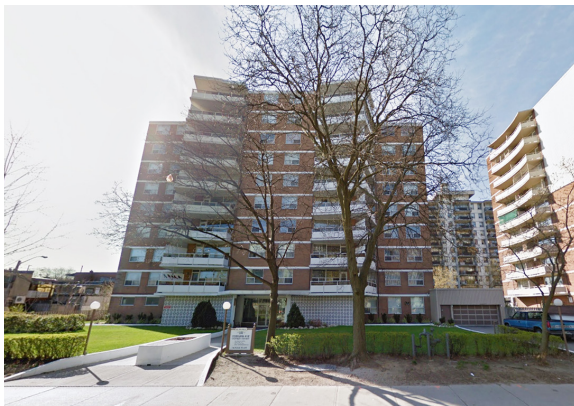
Photo 10: 101 Cosburn Avenue Apartment, West of the TOC Site
