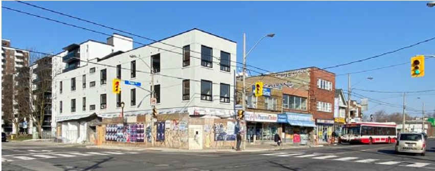
1. North Block: Looking Northwest from Pape Avenue
