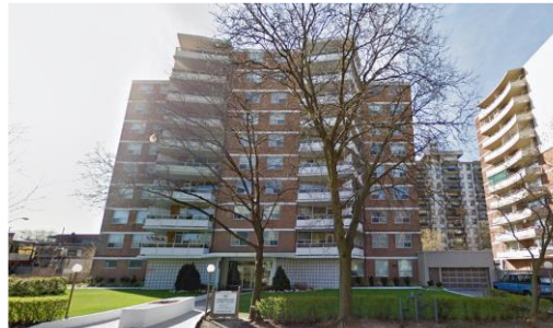
Apartment Building, West of the TOC Site
