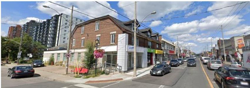
3. South Block: Looking Northwest from Pape Avenue
